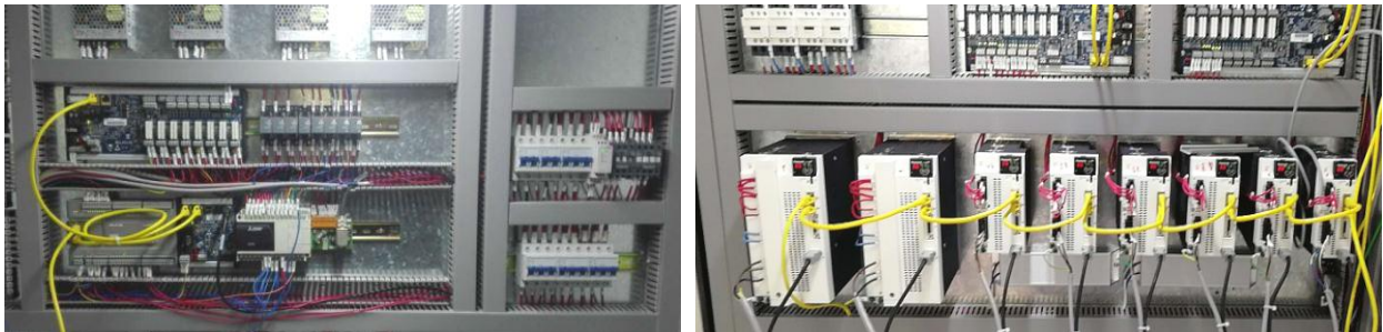
Figure 5-7 Power and signal wiring separation
